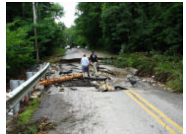
Sucker Brook Bridge Taken By: Liam Powers
